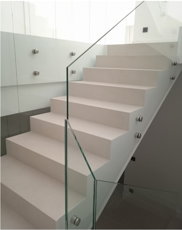
GLASS RAILING WITH SECURIT 10 + 10 GLASS.
