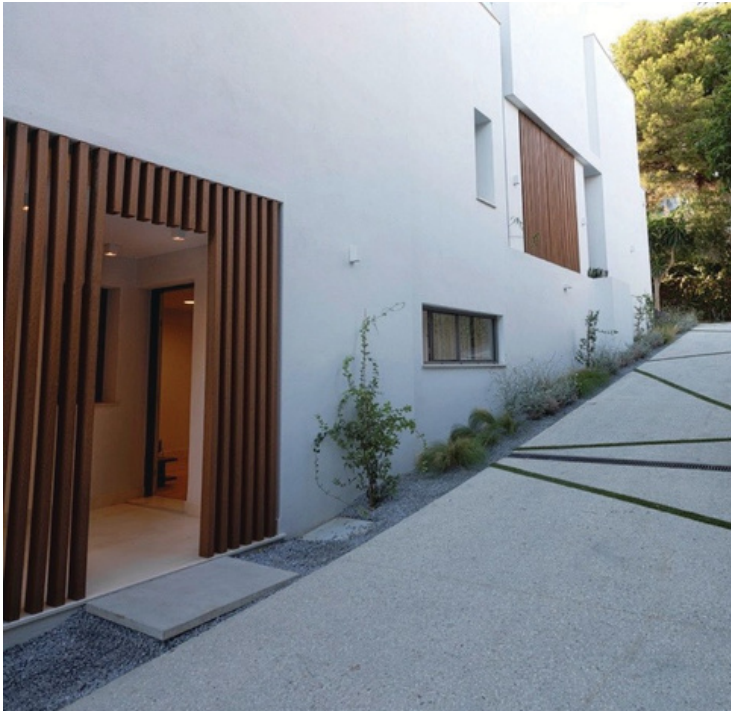
EXCAVATED CONCRETE PAVEMENT AND GRAVEL BEDS
