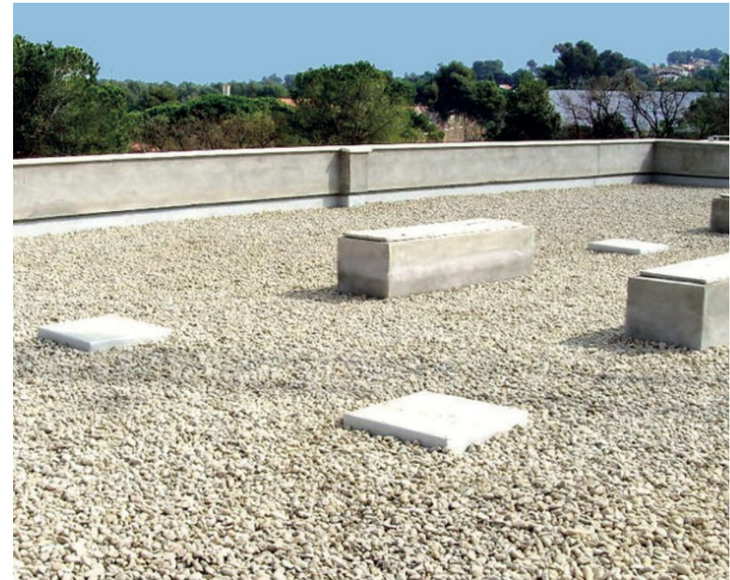
Example of a flat gravel roof
