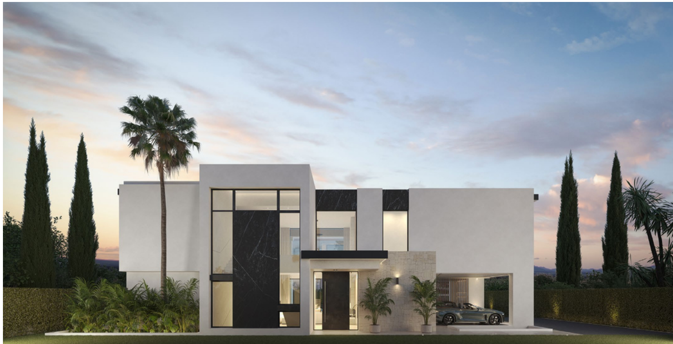
Façade of entrance to the house.
